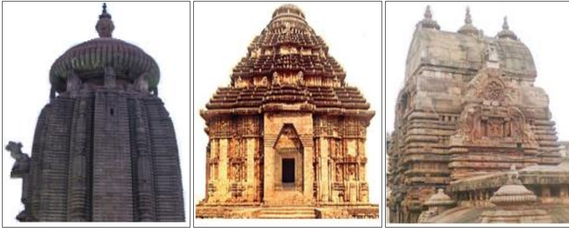
Fig 3a: Lingaraj Temple ( Rekha Deula ) Fig 3b: Konark Temple ( Pidha Deula ) Fig 3c: Baitala Temple ( Khakhara Deula )
